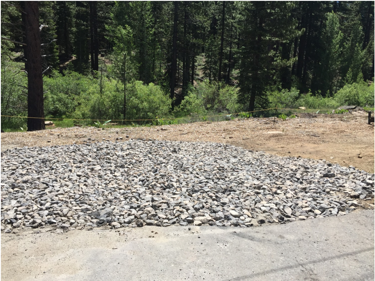
Photo 4: Stabilized entrance to ROW and work area boundary flagging (APM-BIO-26).
